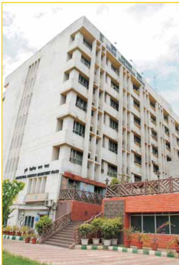
Presently ASRB shares office space in KAB-I building, Pusa Campus, New Delhi
